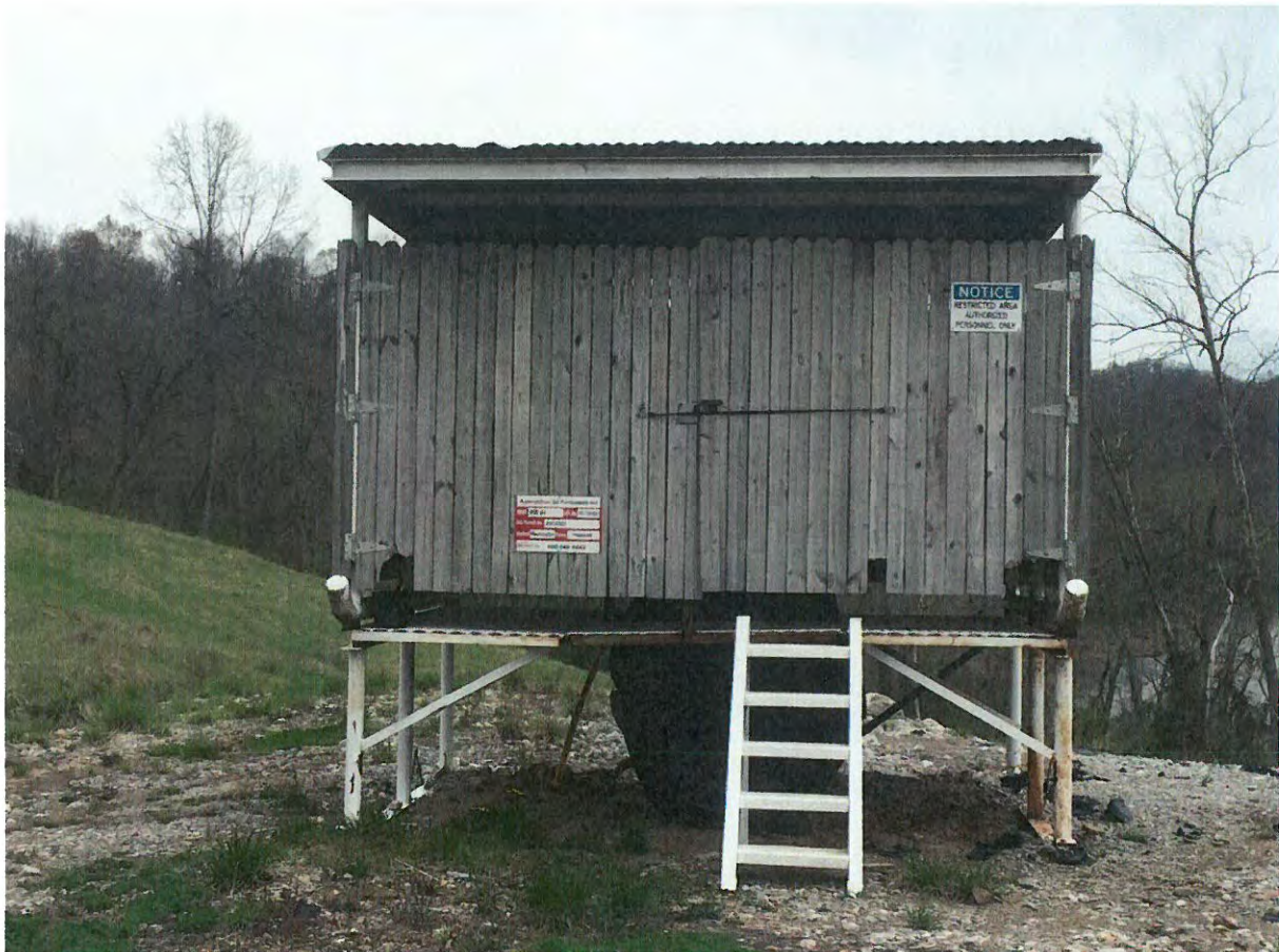
Figure 3 - Locked wellhead enclosure.
