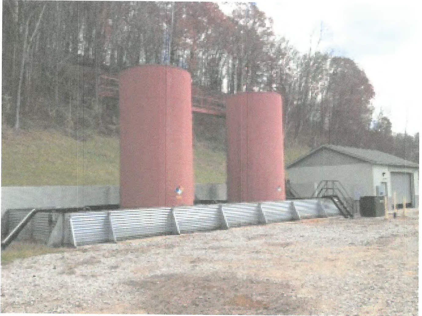
Figure 3 – Photograph of BW#4 Surface Facility.
